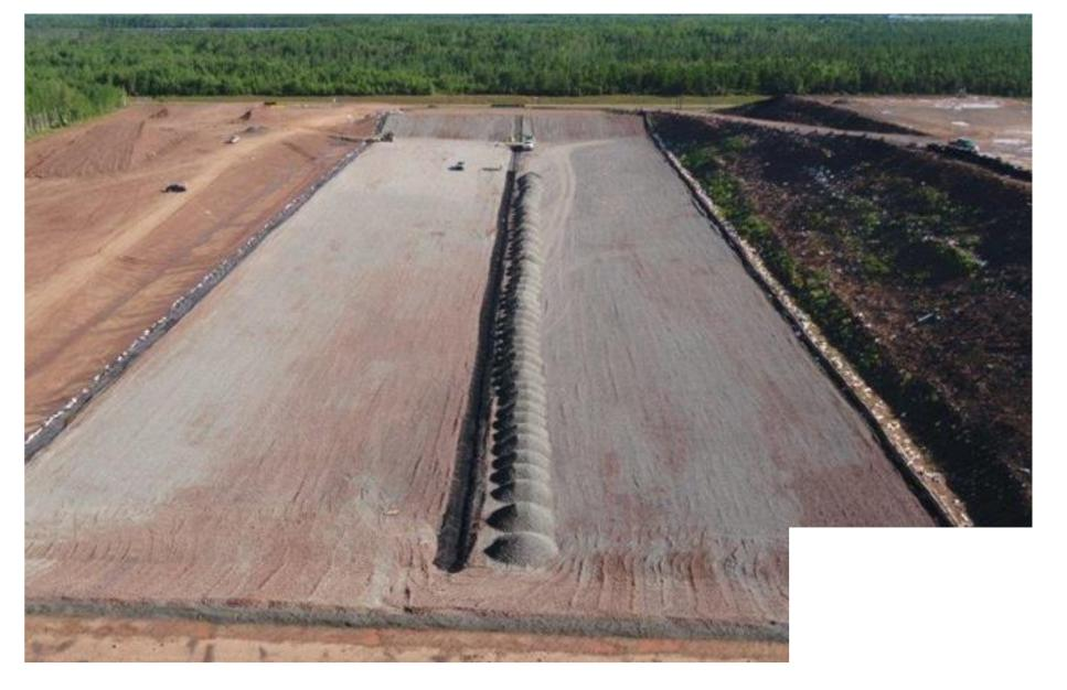
Representative Landfill Construction – Constructed cell essentially complete (some drainage gravel along center line remaining to be spread over central collection pipe (under gravel).
