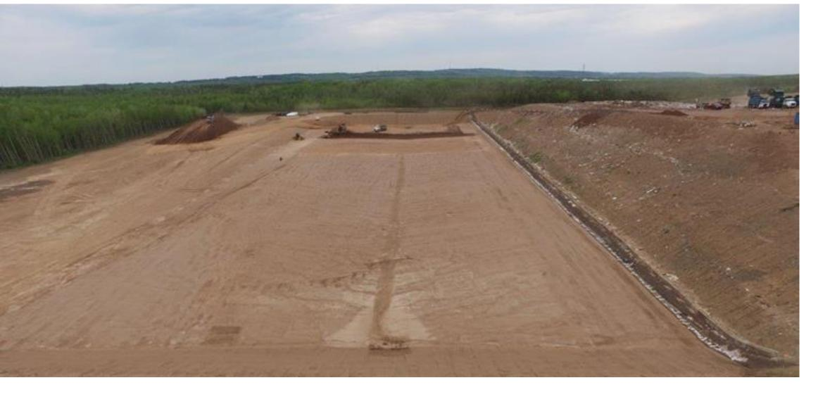
Representative Landfill Construction - Excavate and prepare subgrade (and place underdrain layer, if applicable), place and compact low hydraulic conductivity soil base liner prior to geomembrane liner construction.
